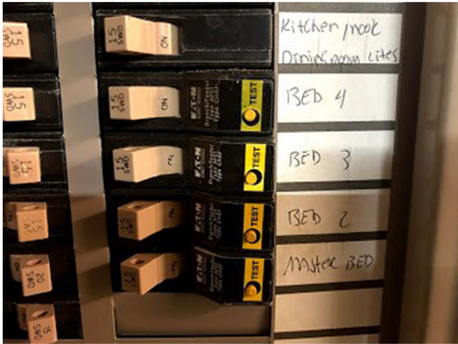
Figure 3. AFCI Circuit Breakers installed in a load center
