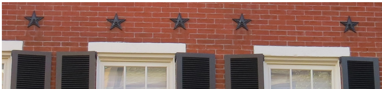
Fig.3- Assortment of anchors, including a star bolt
