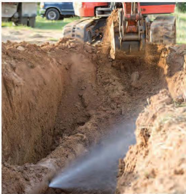
Repairing a water line break
